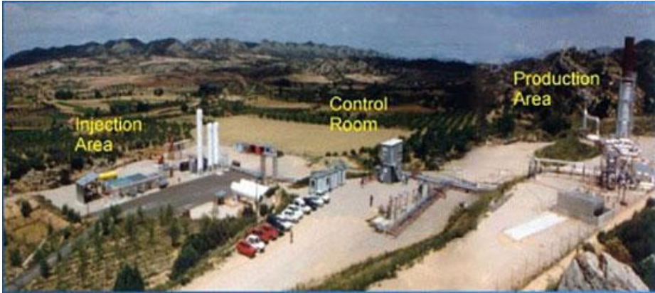
A UCG trial facility at El Tremedal in northeast Spain in 1998
